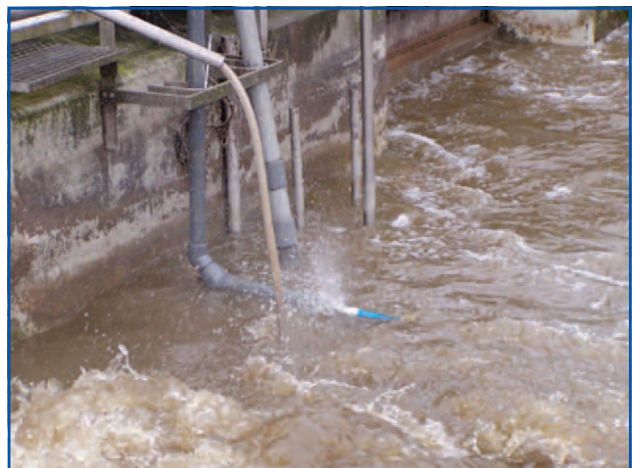
spectro::lyser in aeration tank
