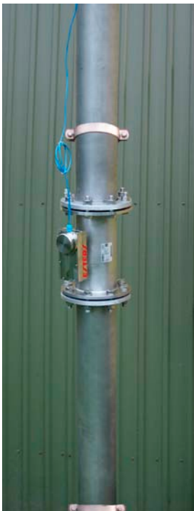
Installation of the GD 300 in a vertically falling line at the fermenter
